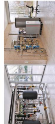
Figure 45. Second stage of the thermodynamic core (left). Heat pump and domestic hot water storage (right).
